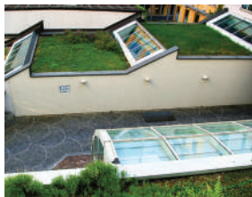
Green Roof System (Atap)
