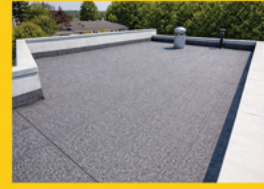
Dak Atap Beton
